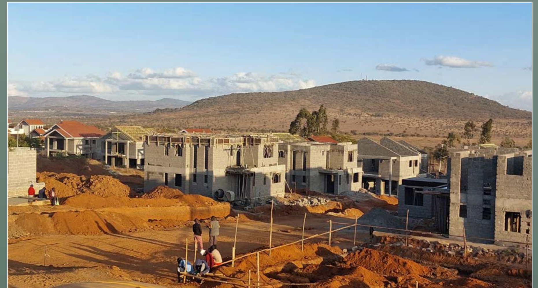
CONSTRUCTION PHOTO TAKEN FROM THE SITE OFFICE, 2023 AUGUST
