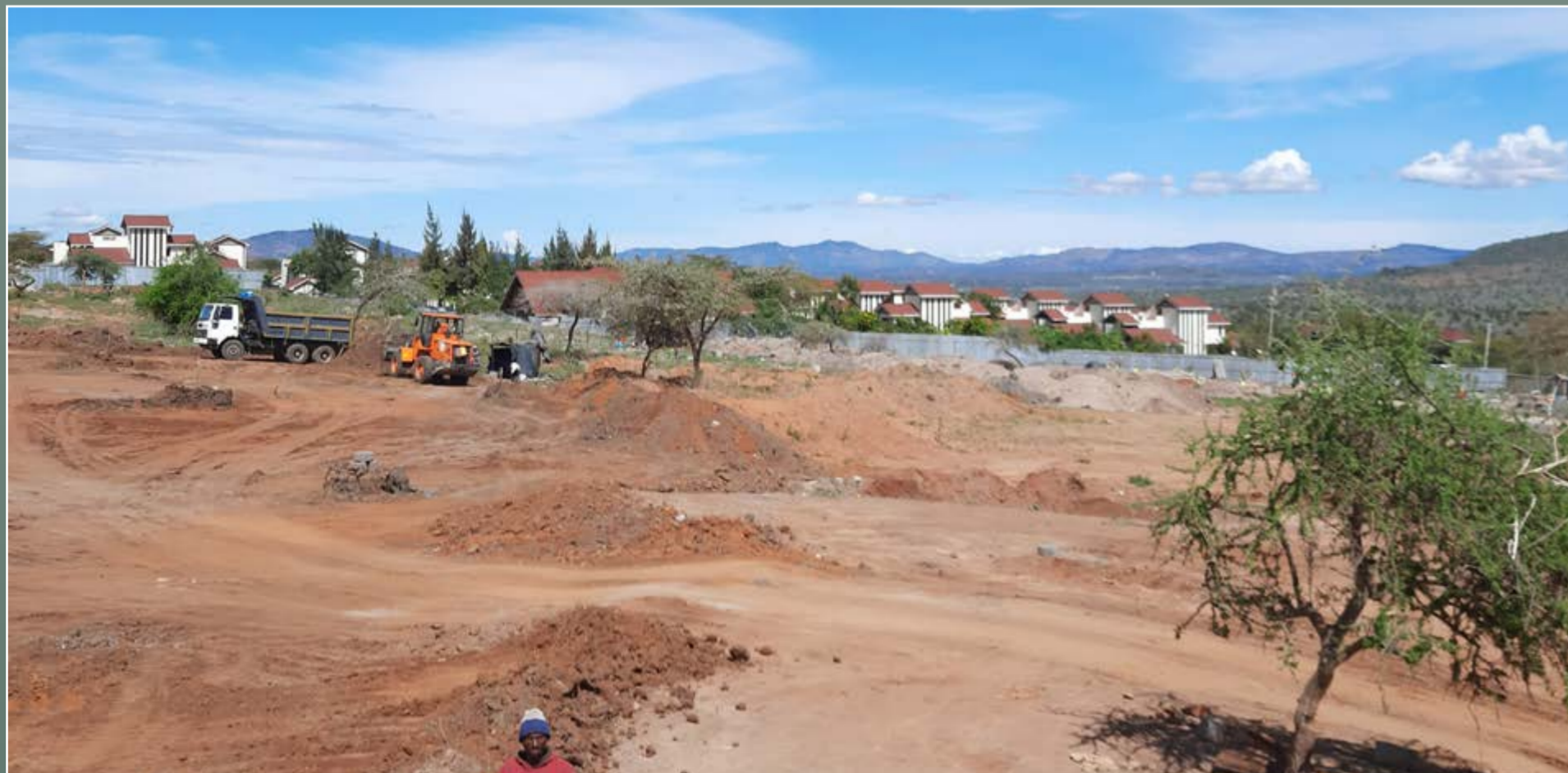
CONSTRUCTION PHOTO OF THE SITE AFTER CLEARING
