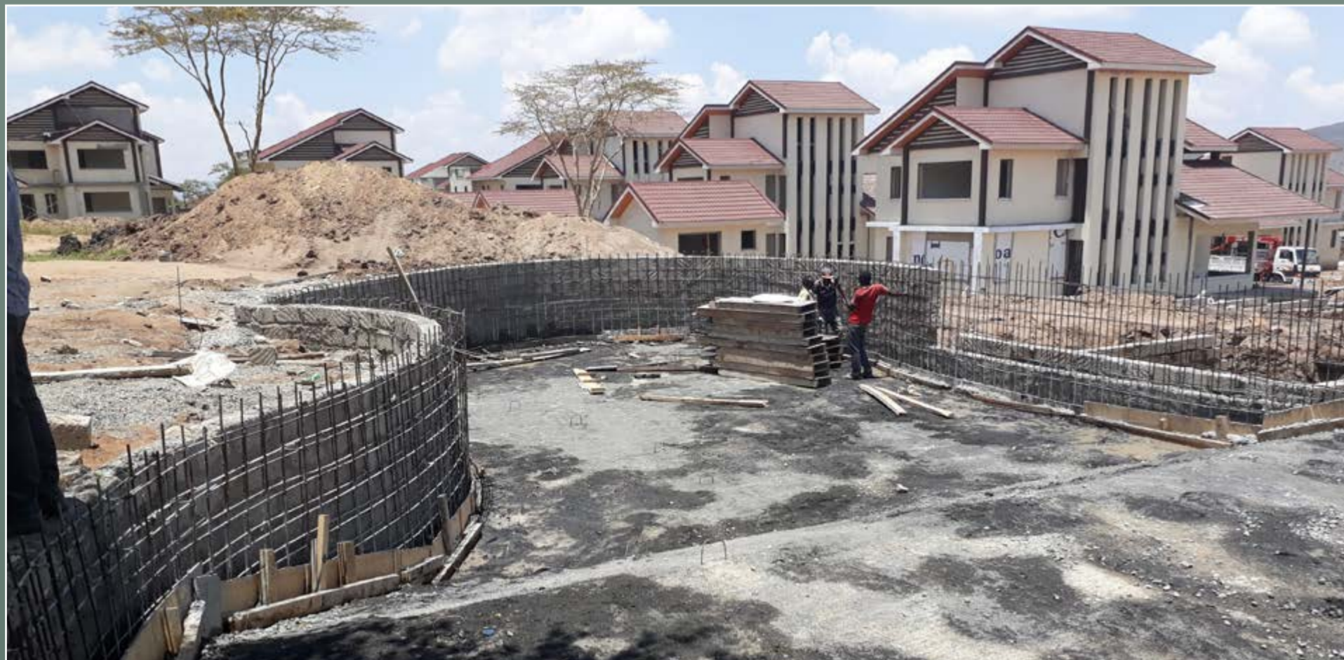
CONSTRUCTION PHOTO OF THE SWIMMING POOL
