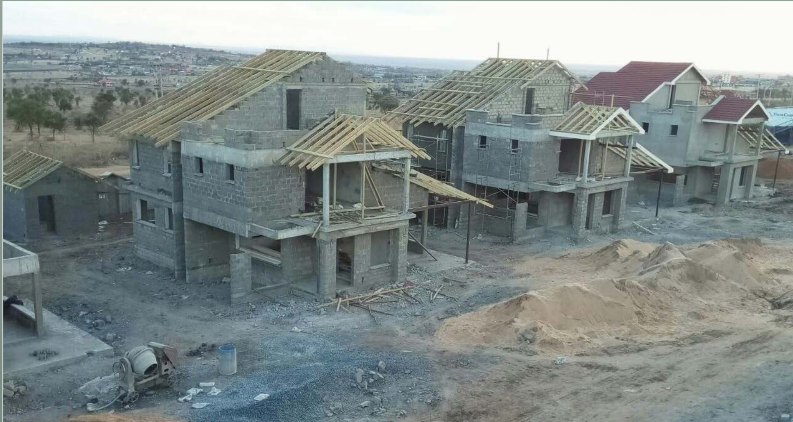
CONSTRUCTION PHOTO OF THE HOUSES
