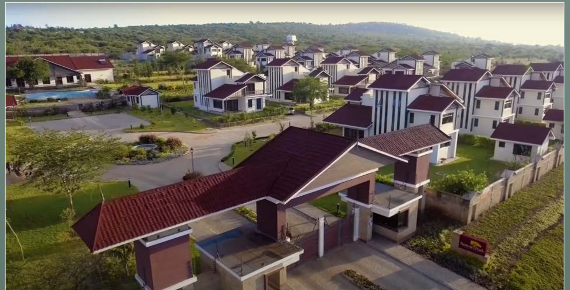
AERIAL SHOT OF THE HOUSES AFTER COMPLETION IN 2017
